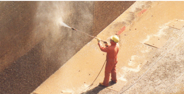
The turbo blaster – a combination of a round-jet and a flat-jet nozzle – removes dirt and paint quickly and effectively.
